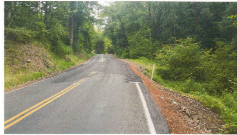
TAKEN ON SOUTHWEST END OF THE PROJECT, LOOKING NORTHEAST
